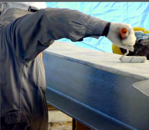
SHOP APPLICATION OF THERMO-LAG 3000. INSTALLATION OF FIBERGLASS MESH REINFORCEMENT
