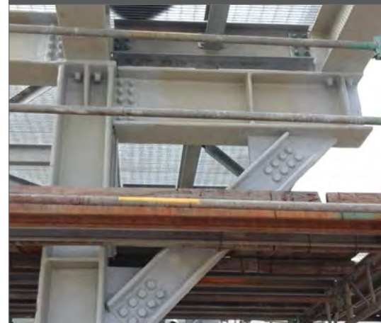
FIELD CONNECTIONS (BLOCK-OUTS) INSTALLED ON-SITE
