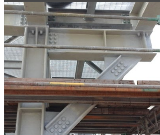
FIELD CONNECTIONS (BLOCK-OUTS) INSTALLED ON-SITE
